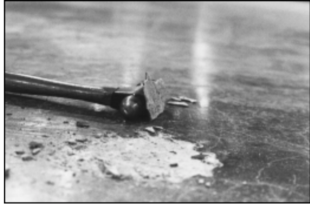
Delaminated Concrete
