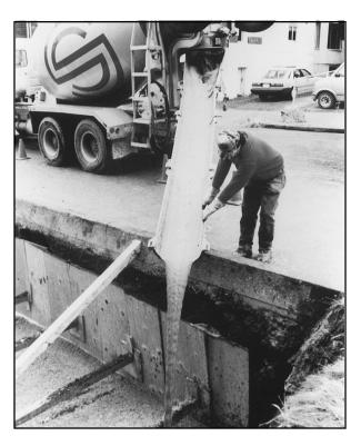
that make best use of economical aggregates, fly ash and other materials. Frequently site-excavated materials and materials that do not meet standards for use in concrete can be incorporated in flowable fill mixtures.
